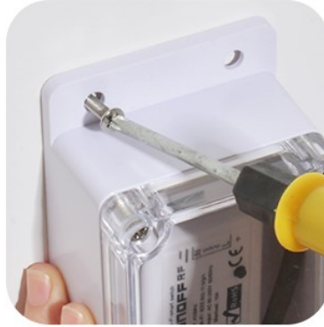
Mount it onto the wall with screws
